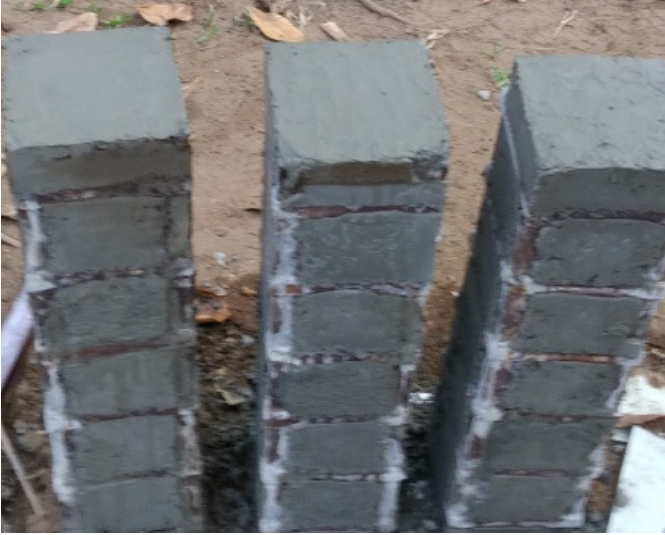
FIG 2 PSC COLUMN AFTER FORMWORK REMOVAL
